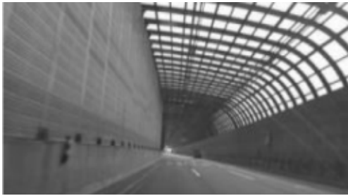
(Central separation wall; closure type)
