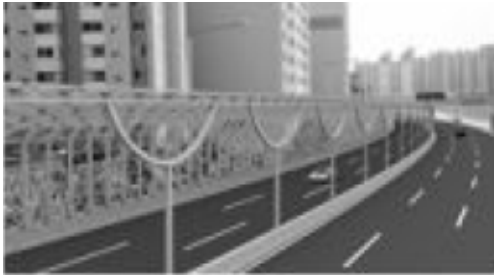
(Half tunnel type; soundproof wall)
