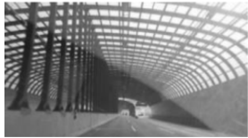
(Central separation wall; open type)
