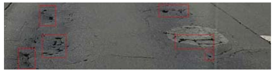
<Fig. 3> Ground Truth Image including Road Damaged Area marked by Red Boxes
