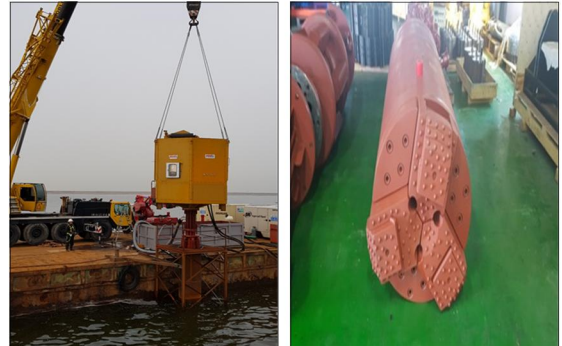
Fig. 13 Excavating equipment : (a) foundation drilling (b) integral type hammer
