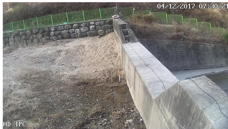
Fig. 3. Panoramic view of the dredged sediment management system in the study area.
