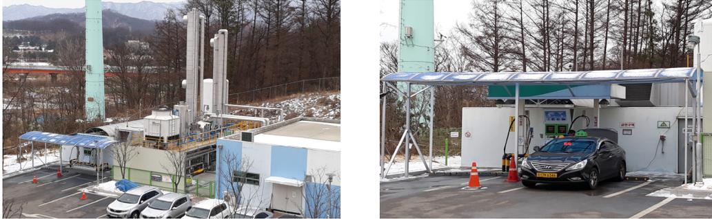
Fig. 4. Whole view of biomethane manufacturing(water scrubbing) facilities and fuel charging stations.
