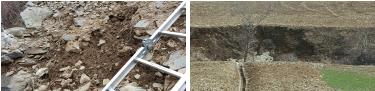
Fig. 8. Pictures of river slope collapse due to rainfall
