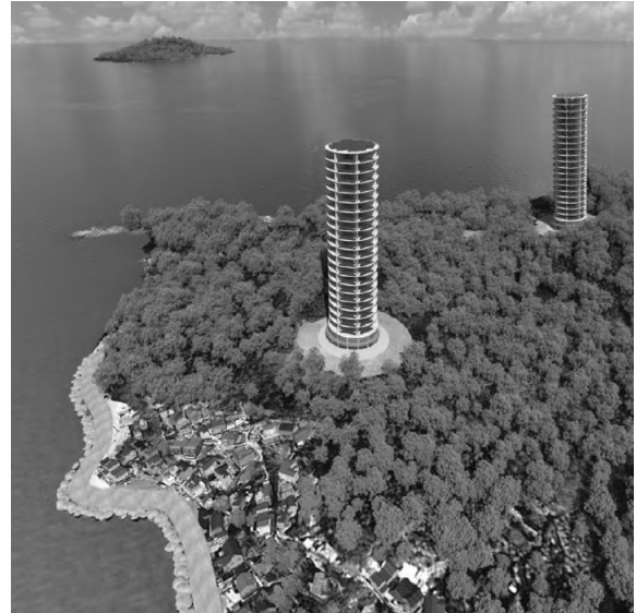
Fig. 1. View of wind power tower with VAWTs
