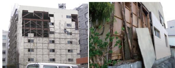
〈Fig. 2〉 Damage of the exterior panels (2011 Tohoku earthquake, Japan)<sup>19)</sup>
