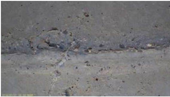
〈Fig. 12〉 Concrete surface image using multi-array camera
