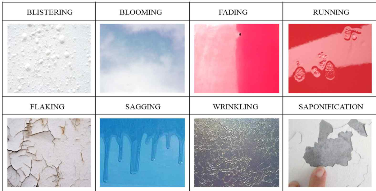
Fig. 3 Common Defects in Paint Works.
