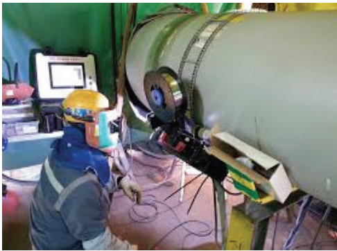
Fig. 1. Example of plant piping inspection using automated equipment.
