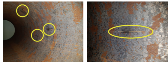
Fig. 12. Mock tubing with random faults.
