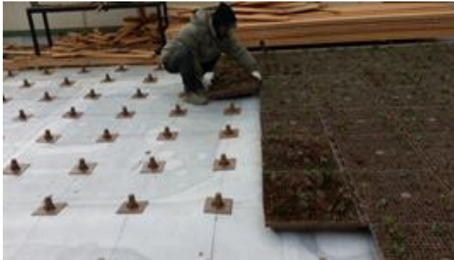
Figure 2. Installation of waterproof sheet and box unit system
