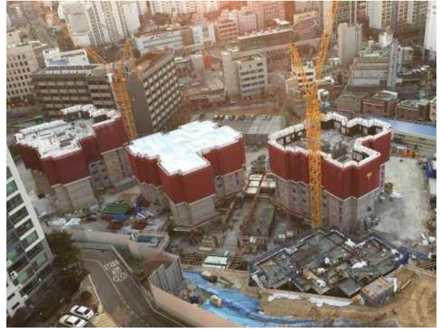
Figure 5. Insulated gang-form keep warming work method
