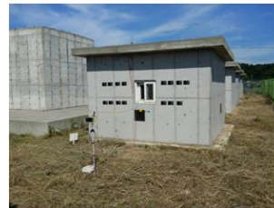
(a) Result of vertical sagging down resistance
