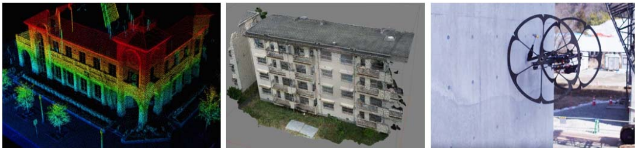
〈Fig. 7〉 Inspection of building using drone
