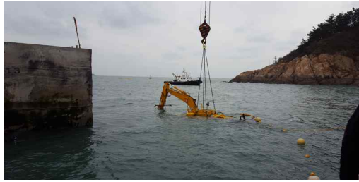
Fig. 15 Robot lowering beside a caisson in Anheung port
