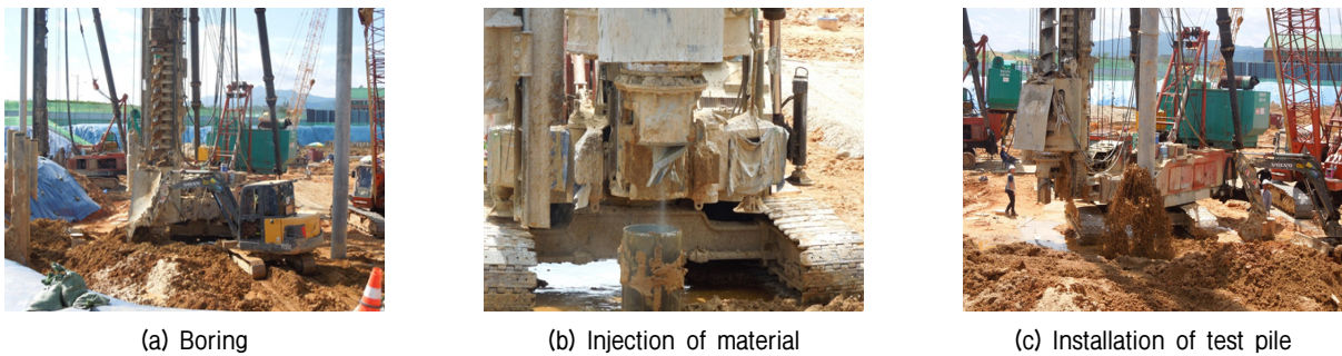
Fig. 6. Process of Installation of test pile
