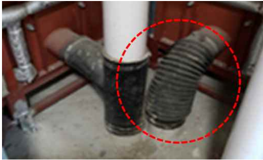
Figure 9. Accessory specialized for connection part of plumbing system
