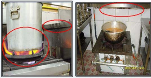
Fig. 2. Damage due to combustion heat
