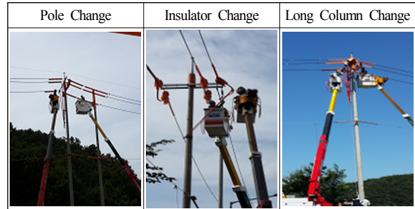
Fig. 16. The demonstration of live-line works.
