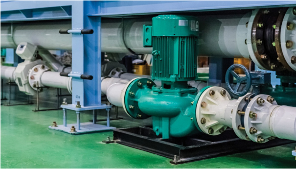
Fig. 7. A photograph of the pump installed underneath the wave flume.
