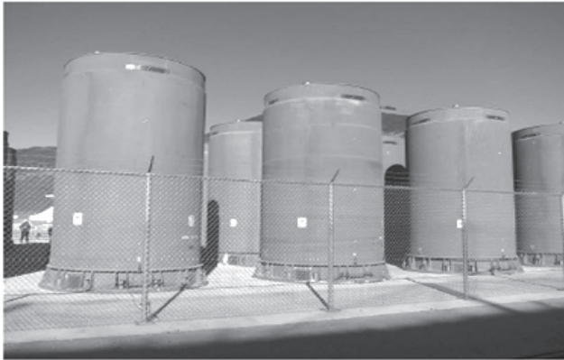
Fig. 4. Holtec HI-STORM dry cask storage systems at Diablo Canyon [77].
