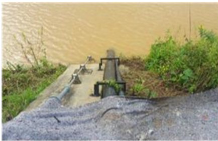
(e) Construction of inflow part
