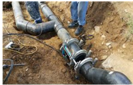
(b) PE water pipe installation
