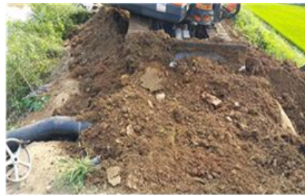
(f) Refilling of dam body
