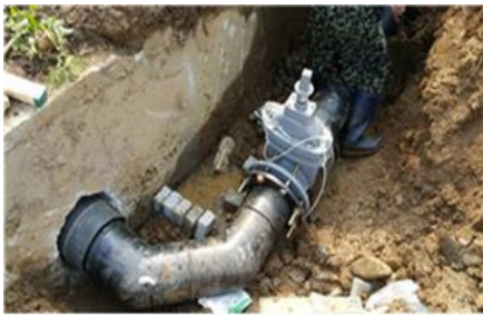
(a) Connection of V-notch part
