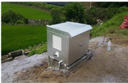
(c) Installation of pump
