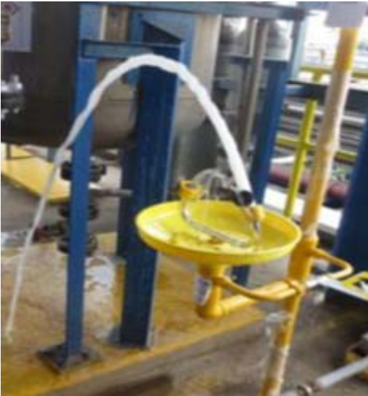
Fig. 6. Inappropriate water height by different pressure resistance.
