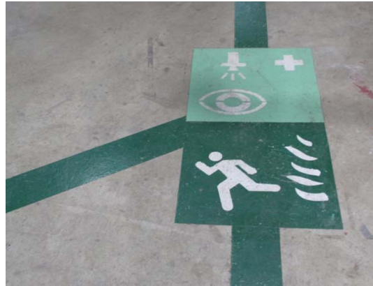
Fig. 3. Route marking to safety shower on floor
