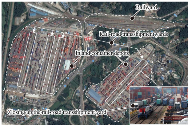
<Figure 1> Top View of the Uiwang ICD and Rail-Road Transshipment Yards (available at http://www.kihoilbo.co.kr/?mod=news&act=articleView&idxno=670311 )
