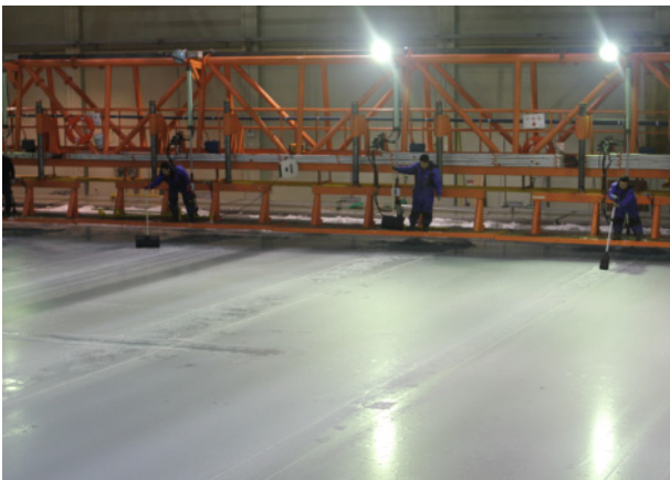
Fig. 3 Broken ice channel preparation procedure
