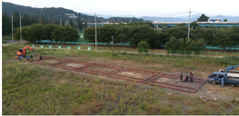
Fig. 4 Foundation of LFR structure
