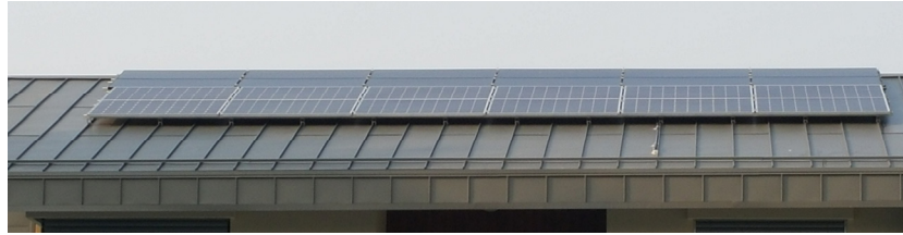
Fig. 1 Installation of rooftop photovoltaic system
