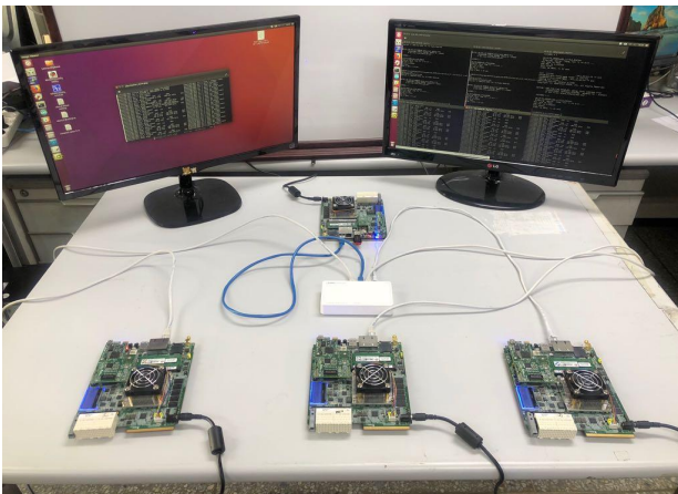
Fig. 6. Examples of IEC 61850 based co-protection system implementation and operational test environment implementation with precision time synchronization.
