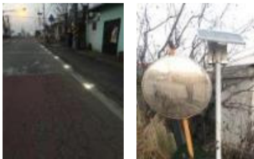
Fig. 10. Improved rural road safety facility 2
