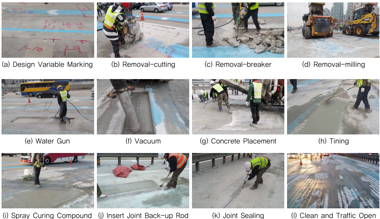
Fig. 3 Experimental Construction Process of Partial Depth Repair
