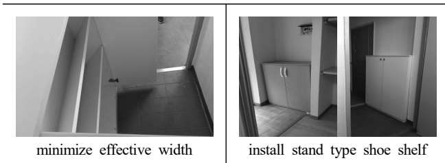
Fig. 7. Improving the installation of shoe shelf
