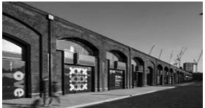
Fig. 6. Transformation of Old Railway Arches, Kings Cross
