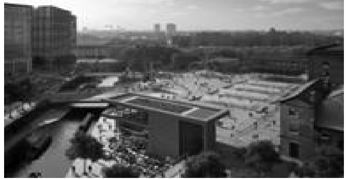
Fig. 5. Elevated View of the 8,000 Square Metre Granary Square, Kings Cross
