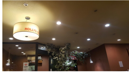
Fig. 7. Plaster board finishing cafe.
