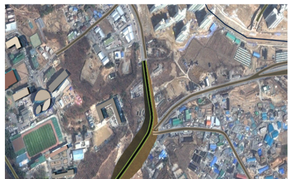
Figure 5. Aerial view of road construction site
