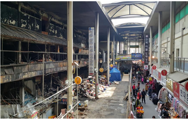
Figure 2. Actual inspection on traditional market.
