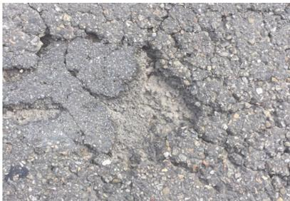
Fig. 2. Shape of Pothole
