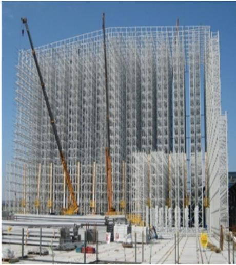
Fig. 1 Structural view of rack type warehouse which is under construction
