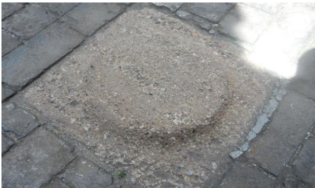
FIGURE VII Monolithic stone base and plinth for a wood column
