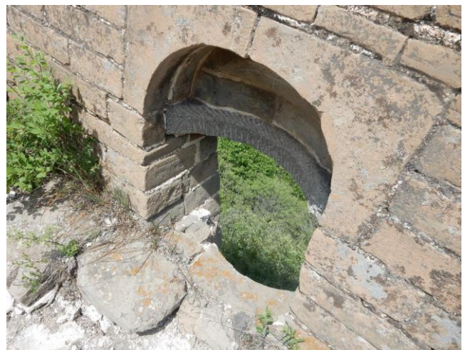
FIGURE VI MATERIAL SELECTION (BRICKS AND GRANITE STONE) FOR THE STONE/SANITARY HOLE OF THE WALL
