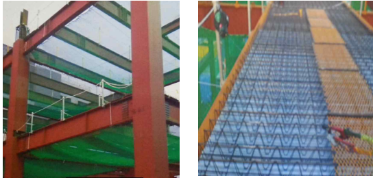
[Figure 14] Deck plate installation after CFT assembly
