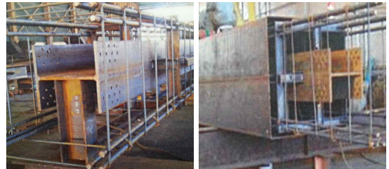
[Figure 12] CFT Reinforcement and formwork installation
