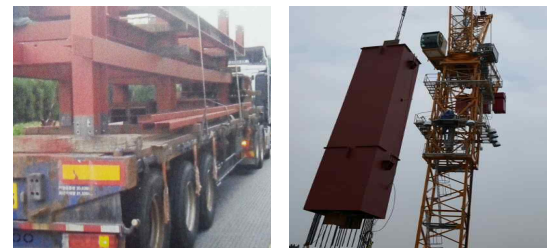
[Figure 13] CFT Transportation and field installation
