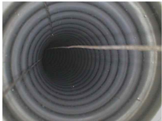
Fig. 3 Inside Image of underground pipe
