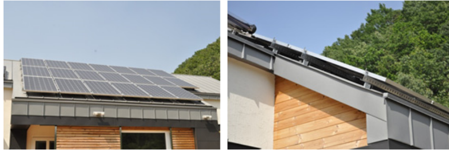
Fig. 2 Semi-integrated with air duct behind
