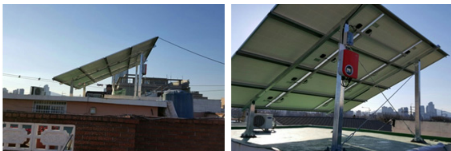
Fig. 1 Mounted modules with air circulation
