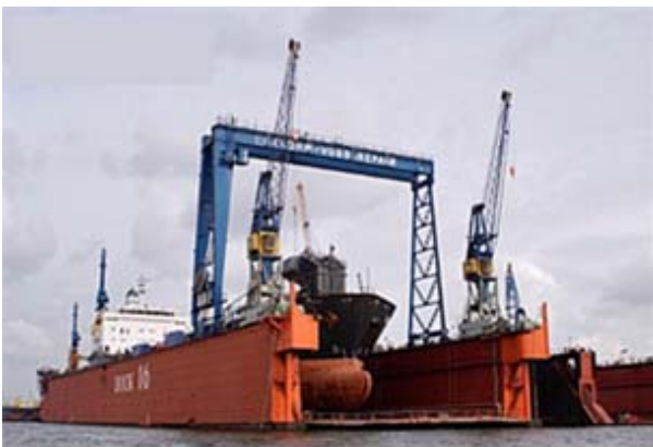
Fig. 2 A floating dock in operation in a ship yard
