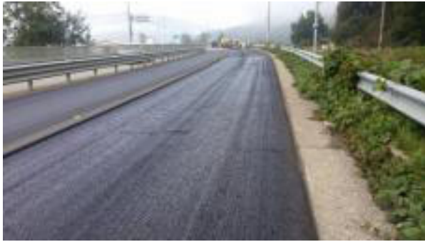
(b) After Sprayed Tack Coat
