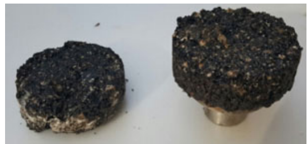
(c) Failure at Tack Coat Layer
