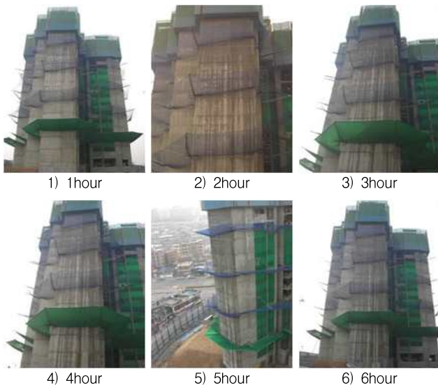
Figure 4. Appearance of moist curing automatic application site
