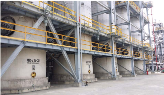
Fig. 5. Reactor of Residue Desulfurization (RDS) Unit.
