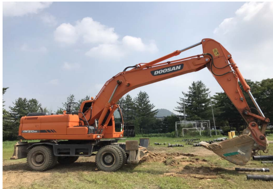
Fig. 2. The picture of a 21 tons of Excavator.
