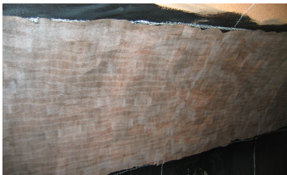
Fig. 6. Surface condition after cleaning
