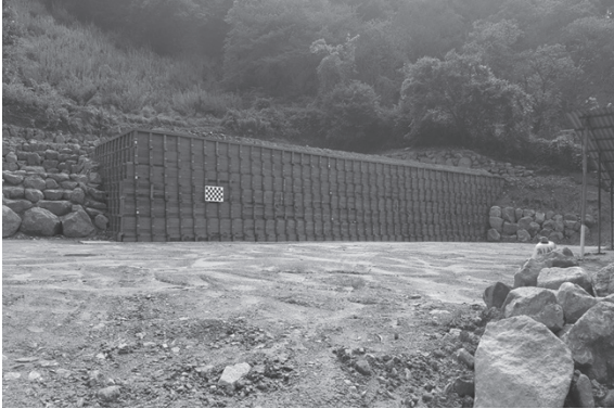
Fig. 3. Real form of the reinforced-soil wall
