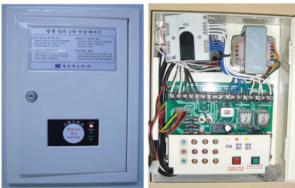
Figure 2. Fire shutter's interlocking system.
